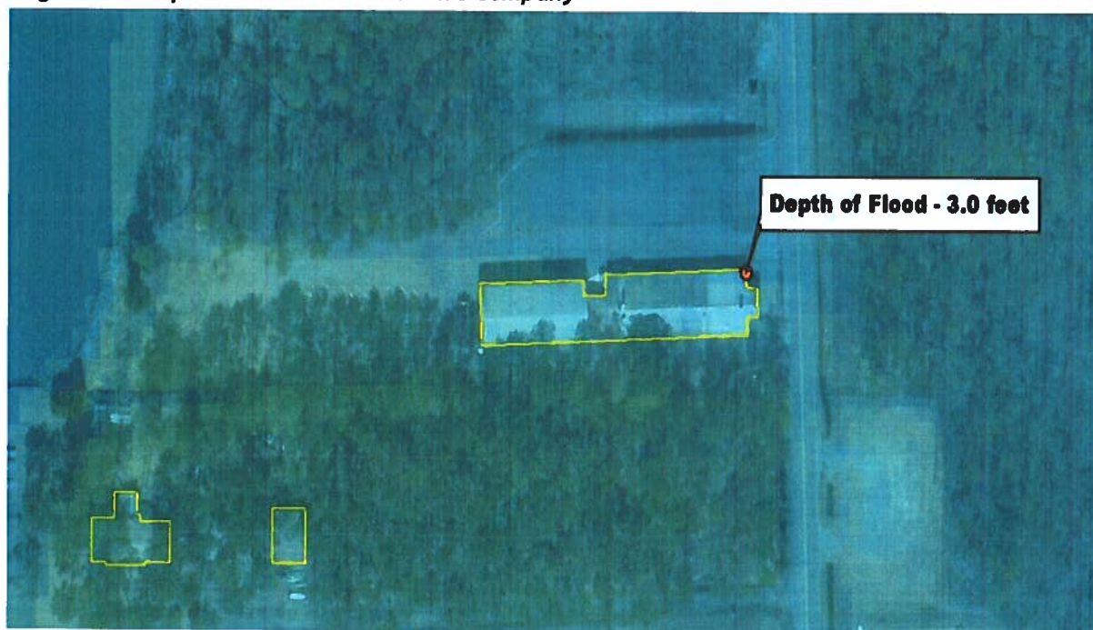
Figure 9 - Hooper's Island Volunteer Fire Company
